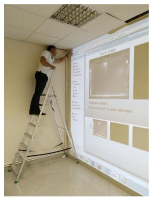
Pic. 16 Calibrating the upper left corner (wall)
